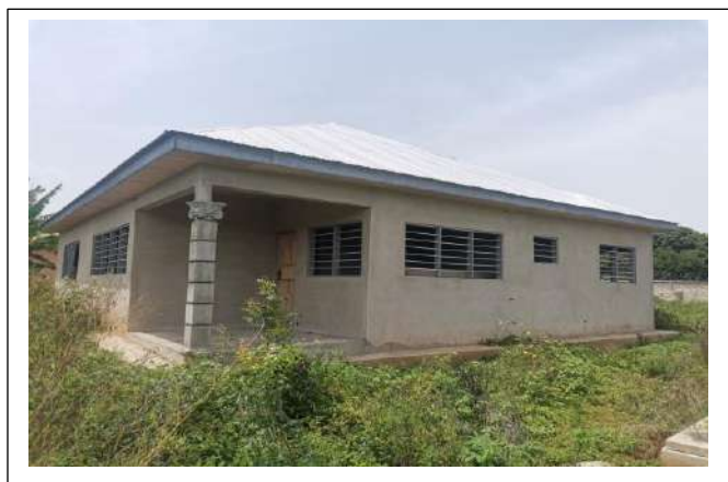
Construction of shelter home at Tokor
