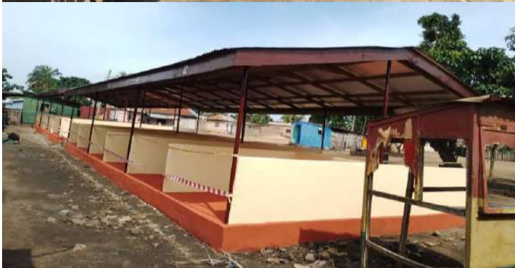
Renovation of Avoeme market shed
