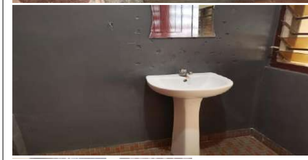
Office washrooms and drainage system were renovated
