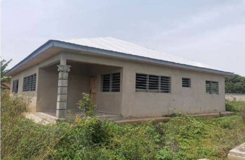
Construction of shelter home at Tokor
