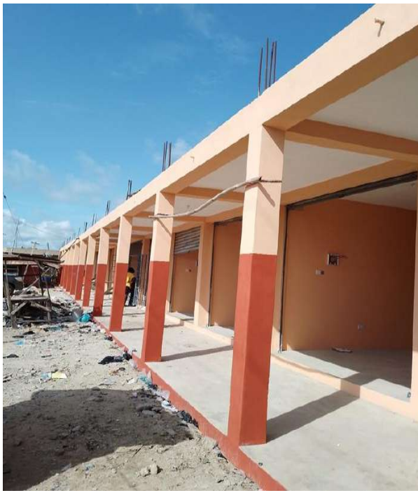
Completion of 20-unit lockable market stores at Denu market
