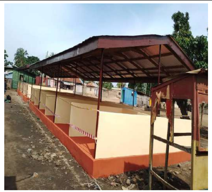
Aflao- Avoeme Market Shed renovated
