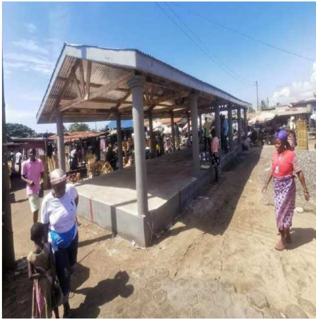
Completion of 1No. Market Shed at Aflao Market
