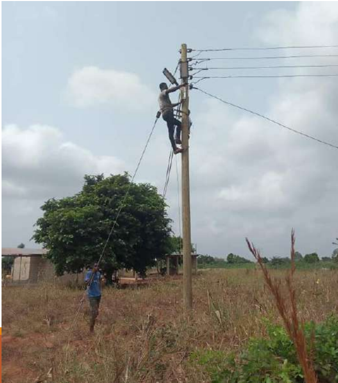
Procurement and installation of 300 streetlights
