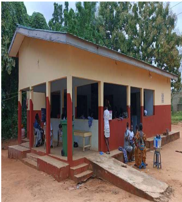
Completion of CHPS compound at Wudoaba
