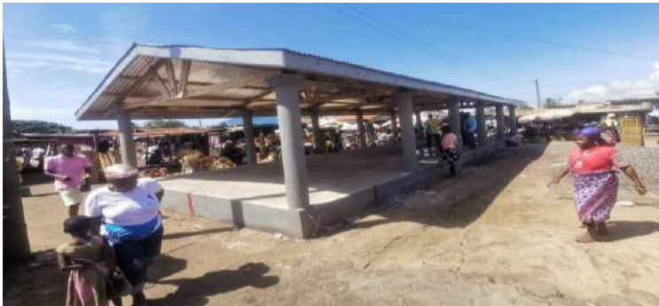
Construction of 1No. market shed at Aflao market
