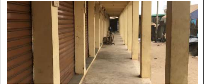
Completion of 28-unit lockable market stores at Aflao Lorry Park
