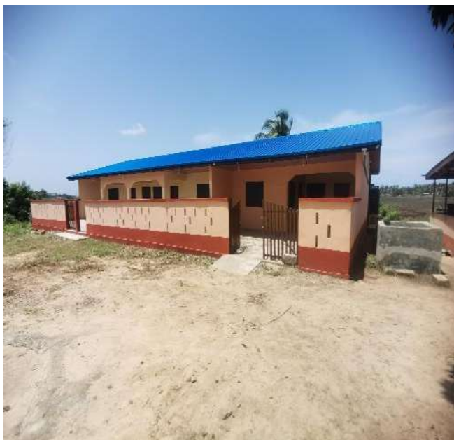
Completion of CHPS Compound at Wudoaba
