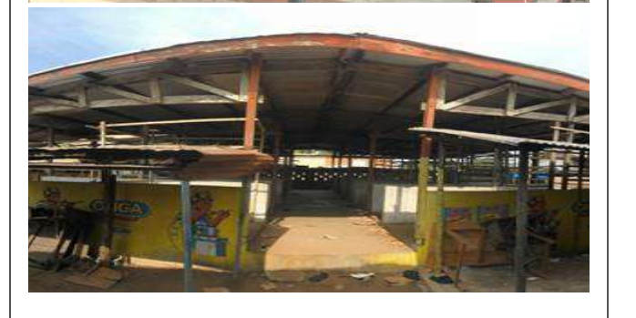
Denu market sheds renovated
