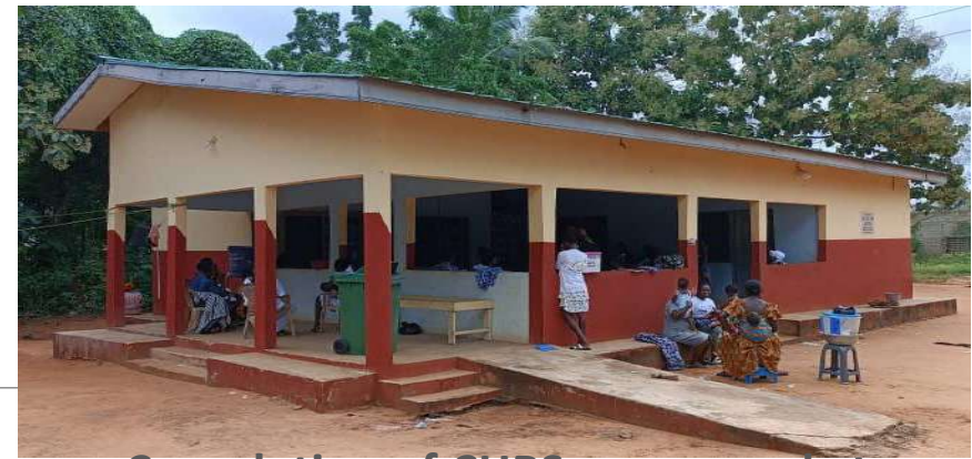
Completion of CHPS compound at Wudoaba
